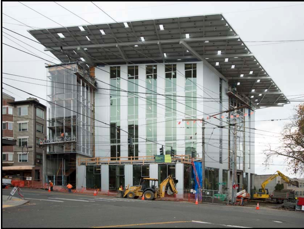
Figure 3. The Bullitt Center – note the prominent roof top solar array and the “Irresistible Stair” in the light filled stairwell (left). Photo by John Stamets
